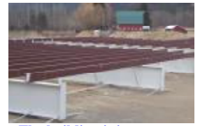
The building is in progress
